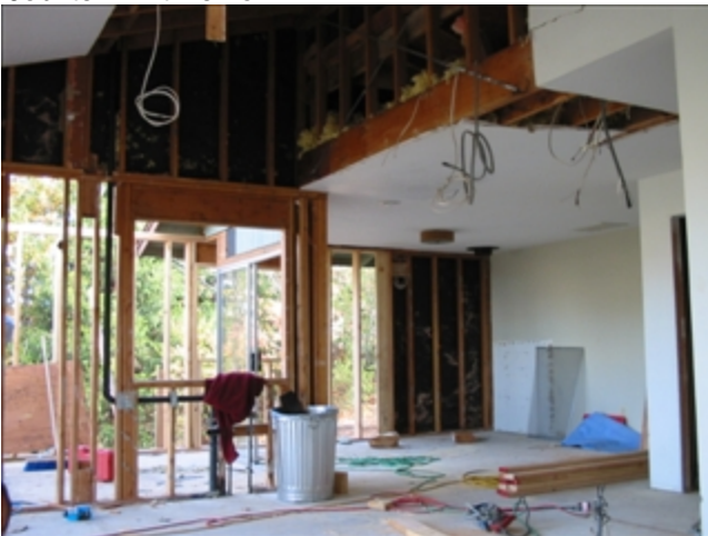
After demo, framing started
