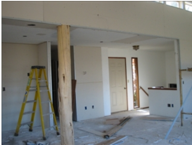
Ready for taping.
